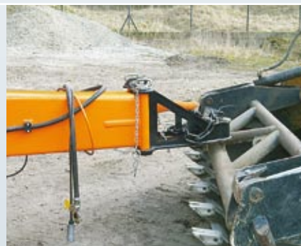
Displacing the machine by wheel loader
